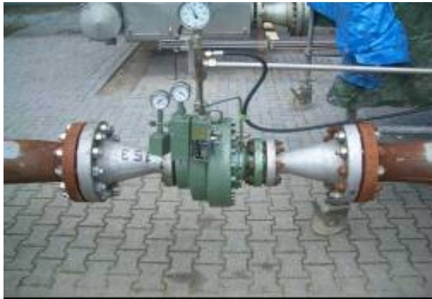
a) Regulator without sound damper
